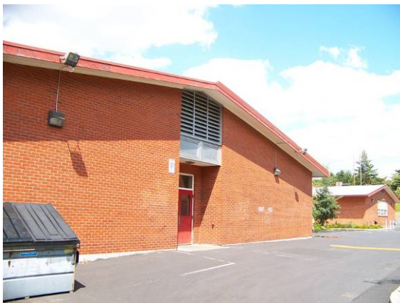
Main building (176A), south (rear) elevation, looking northeast.
