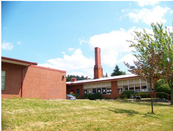
Main building (176A), west (side) elevation looking southeast.
