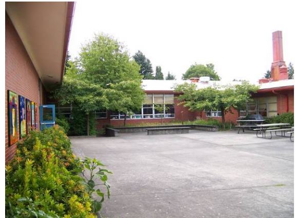
Main building (176A), courtyard, looking southwest.
